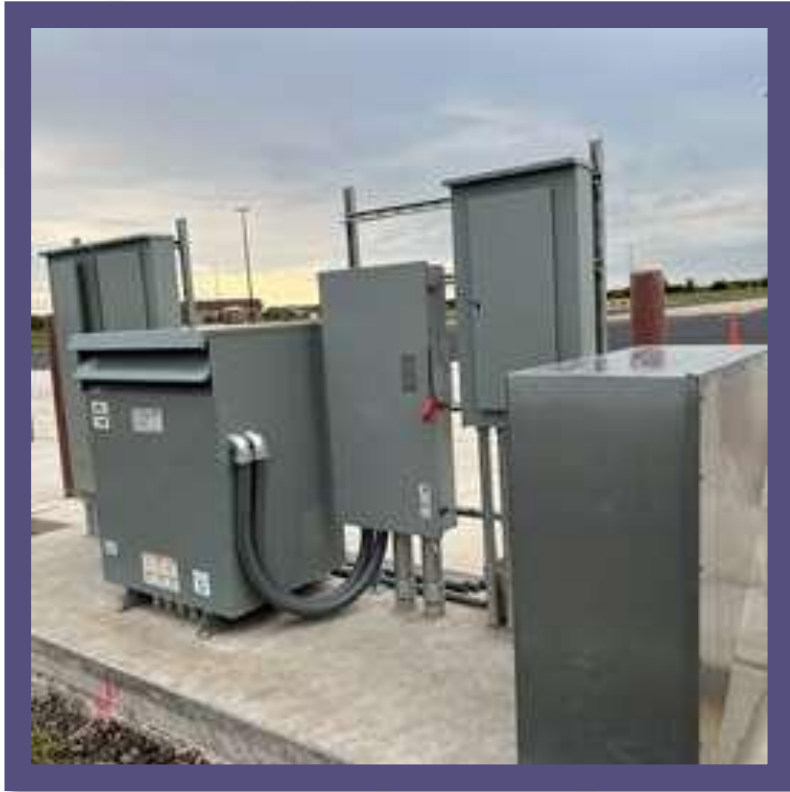
Transformer Switchgear Main Distribution Panel
